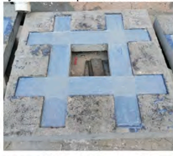
Slab strengthening by NSM technique by adding a layer of concrete.
