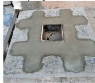
Slab strengthening by NSM technique by adding a layer of concrete.
