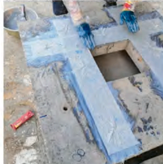
Slab strengthening by EBR technique with anchors.
