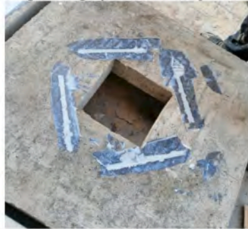
Slab strengthening by EBR technique with rods at the corners of the opening.
