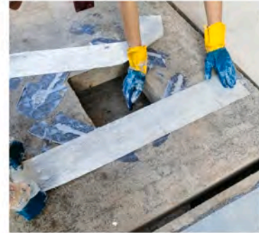
Slab strengthening by EBR technique with rods at the corners of the opening.
