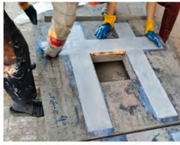
Slab strengthening by EBR technique without anchors.
